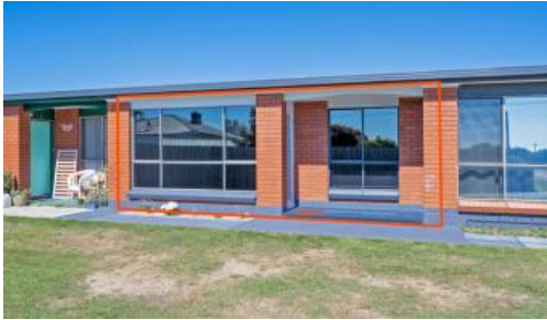
Unit 2/2 Lowe St, Wynyard
