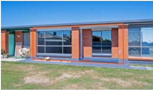
Unit 2/2 Lowe St, Wynyard
